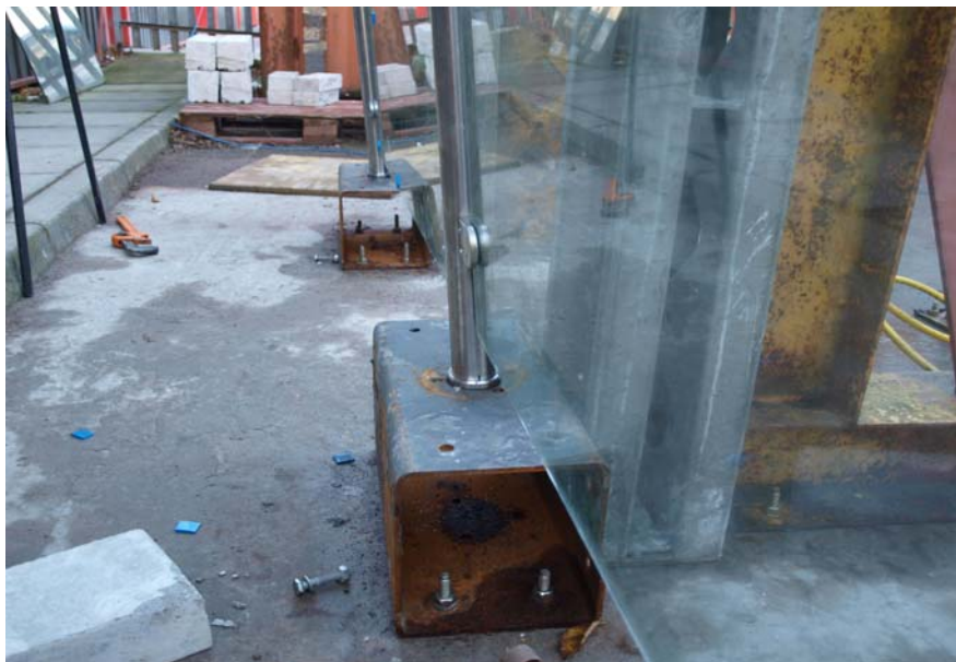
Photograph 2: Method of fixing balustrades to test slab.
