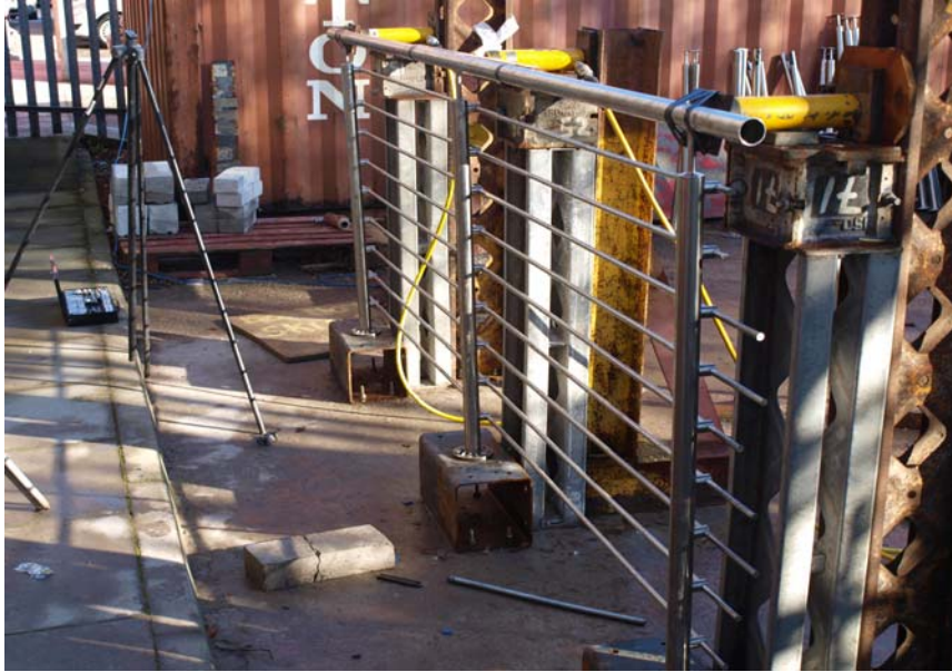
Photograph 3: Load testing of balustrade system with metal rod infill panels.
